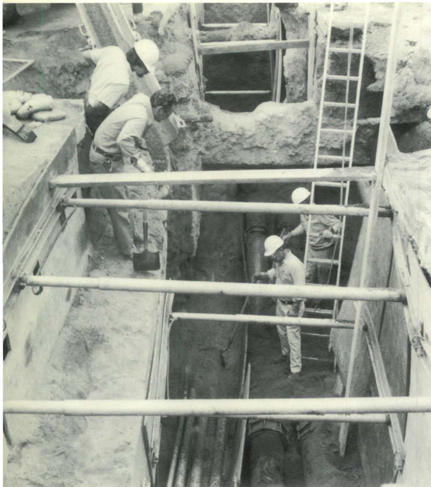
ABOVE: To provide clearance for a new Pasadena city storm drain, the Plant Maintenance staff excavates and lowers 14 underground conduits containing much of the College's communication lines and chill water ducts.
